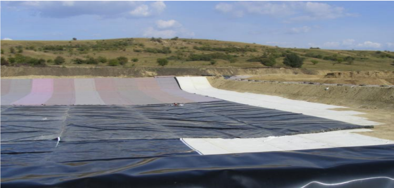
Fig.2.2. Isolation system of a future landfill with geomembrane
