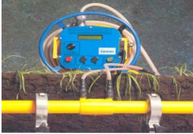
Figure 6 . Electro - fusion Welding Method
