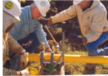
Figure 7. Butt-welding method
