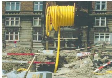
Figure 21 . Laying pipes in trenches easily
